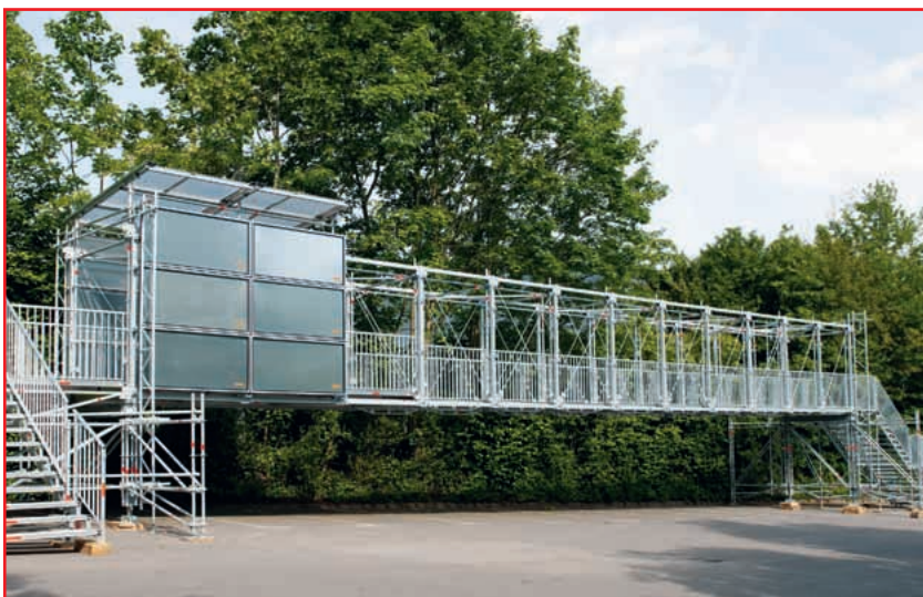
In use as a footbridge, span about 25 m, with Protect cladding and roofing in places
