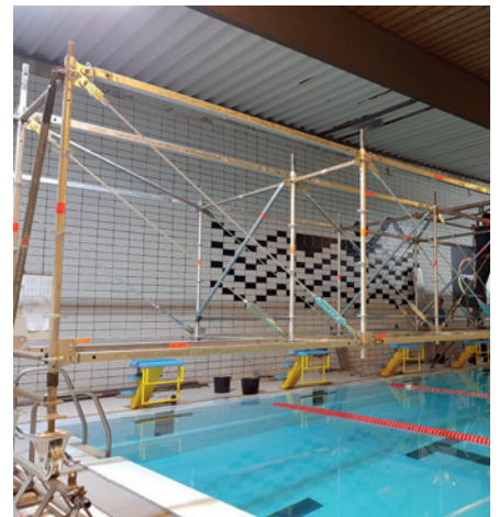
Mobile ceiling work scaffolding over a swimming pool
