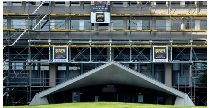
Allround Bridging System for support of facade scaffolding above a projecting roof
