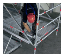
Cantilever method of bridging using Allround FW System
