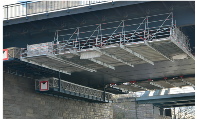
Aluminium FlexBeam as work scaffolding underneath a motorway bridge
