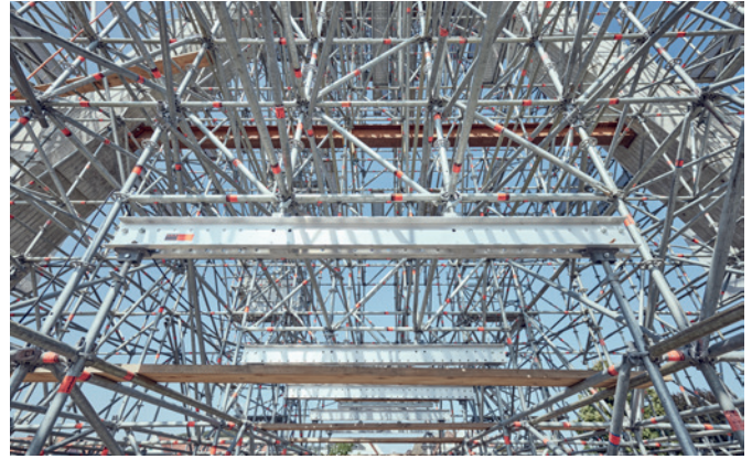
Aluminium TwixBeam in a birdcage scaffolding of a bridge tower
