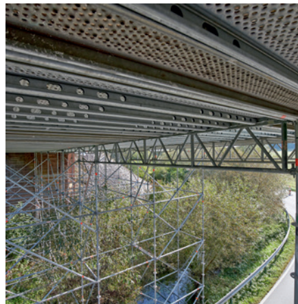
Allround lattice beams with wedge heads
