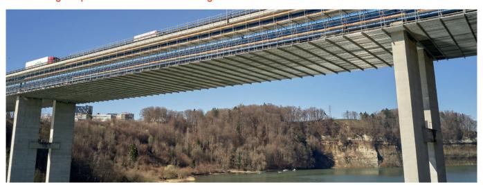
Using the cantilever method for the FlexBeam aluminium U-beam, U-FlexBeams can be used to assemble surface scaffolding underneath a bridge – incrementally, quickly, without improvisation and more safely too. To do so, only three components are needed as tools – the roller unit, the receiving bracket and the fitting retainer.
