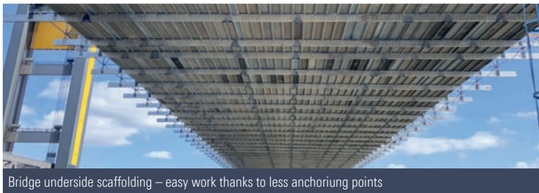
FlexBeam as birdcage scaffolding
