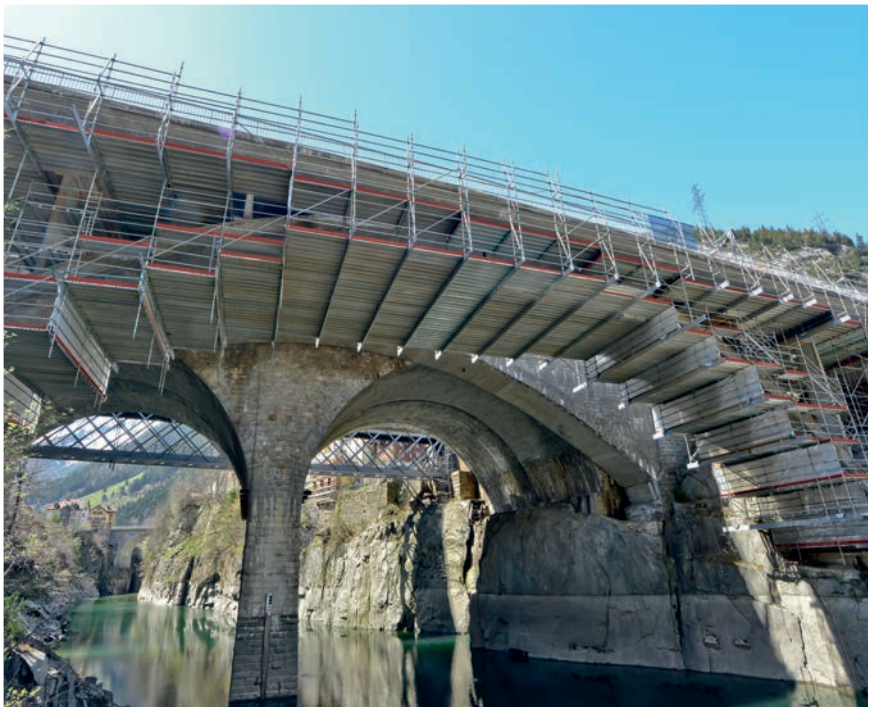
FlexBeam dimensionally and structurally integrated into Allround Scaffolding
