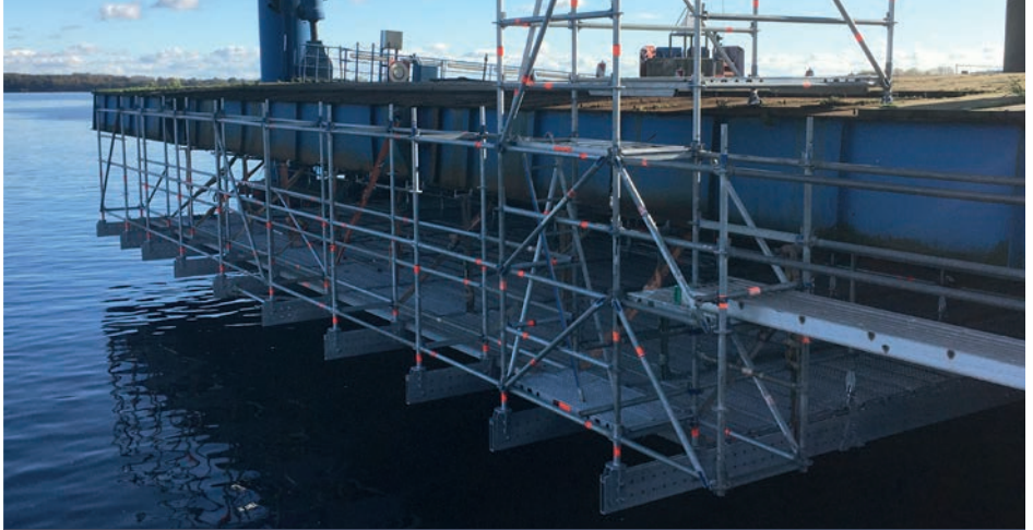
FlexBeam as surface scaffolding at a shipping pier
