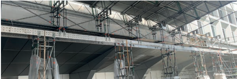
Support for cassette roof – to open the grid dimensions of roof and support structure
