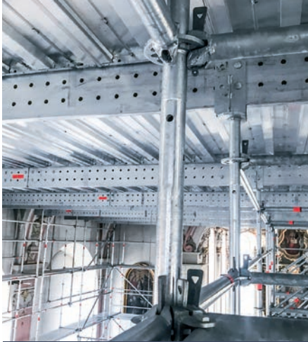
FlexBeam as birdcage scaffolding
