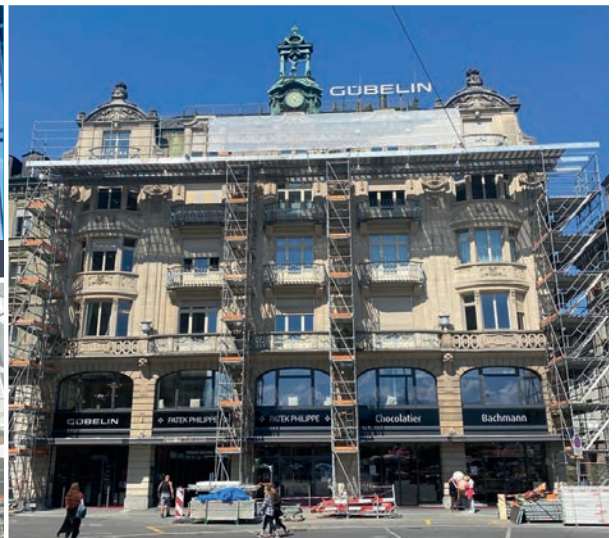
Work platform with material-saving scaffolding structure
