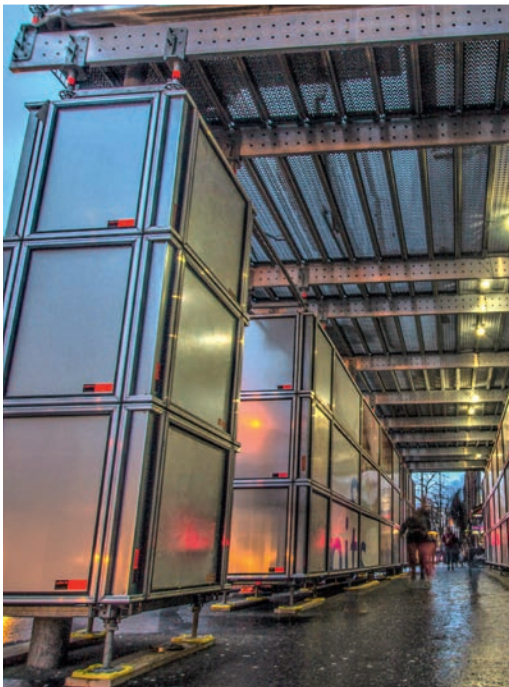
FlexBeam in combination with Protect System as walkway with more than 1.50 m width
