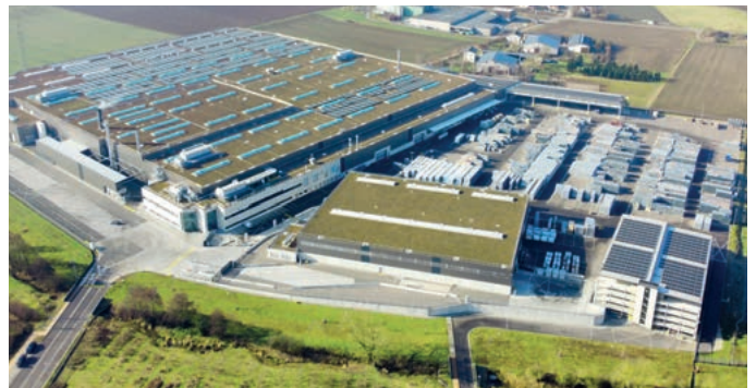
Plant 3 in Cleebronn
